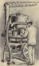
FILLING BY MACHINERY
